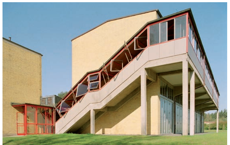
9. School-building after restoration, 2007. BRENNE Gesellschaft von Architekten mbH, Berlin
