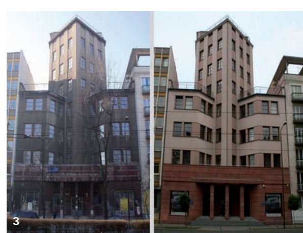
3. Building of General Mutual Insurance Company in Łódź, arch. Waclaw Rytzel, 1929. Photo by authors, 2003, 2009
