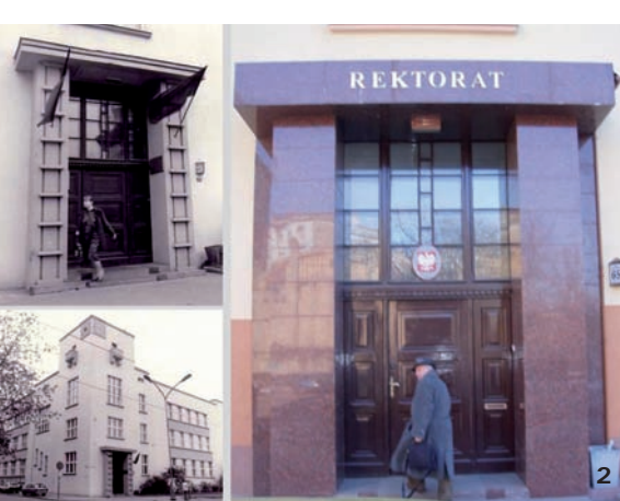
2. Division of Sewerage and Water Magistrature of Łódź, architect Wiesław Lisowski, (1927) 1928. Photo by authors, 1985, 2009
