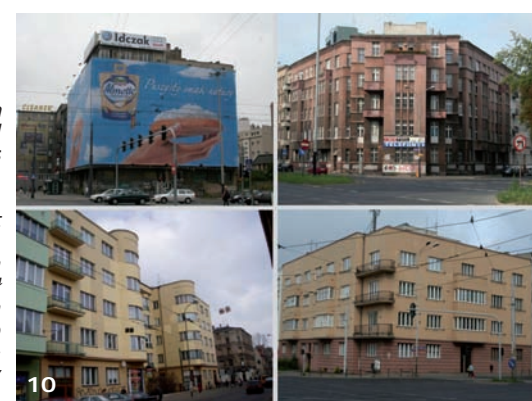
10. Łódź townhouses, corner at the intersection of T. Kościuszki and A. Mickiewicza avenues architect unidentified; Uniwersytecka and St. Jaracza streets, architect Paweł Rudolf Sunderland 1928; Zielona and Gdańska streets, architect Paweł Lewy 1936; G. Narutowicza and St. Kopcińskiego streets, architect unidentified. Photo by authors, 2009
