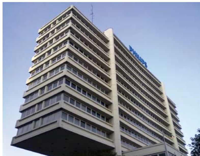
6. Vienna, Philips House, former headquarters of Philips Austria, Triester Straße 64, arch. Karl Schwanzer, 1965 (photo Wolfgang H. Salcher)
