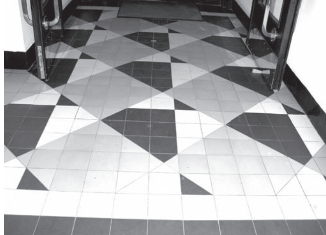
3. Gdynia Port Authority S.A. (former Customs House), by architect Stanisław Odyniec-Dobrowolski (1934-1936) – fragment of the preserved mosaic floor of the vestibule (three-colour, diagonal geometric composition). Photo by A. Orchowska-Smolińska
