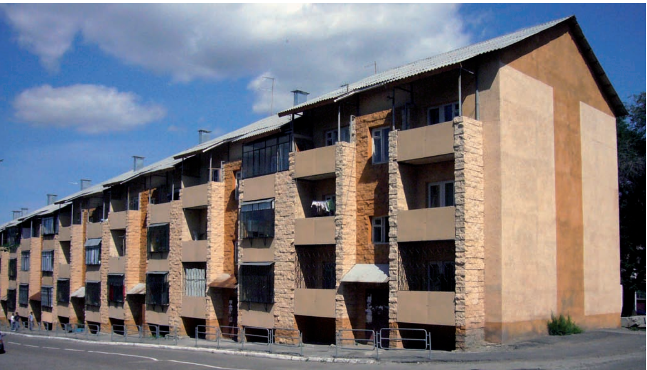
8. The building was bought by a private investor and subsequently redecorated; balconies were added and the façades had natural stone cladding and were painted. Photo by the author
