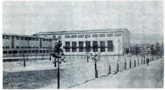
13. Photo of the school and kindergarten complex published by Borngräber and Pistorius/ Schädlich as a 1934 photo
