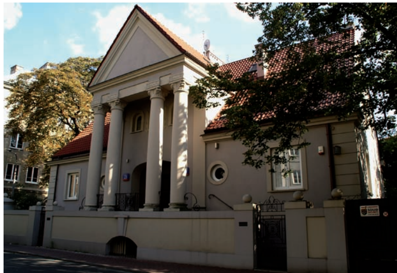
3. Repeatable semi-detached house in 23/25 Mochneckiego St., Warsaw, designed by arch. Romuald Miller, 1924. Photo by J. Roguska, 2009
