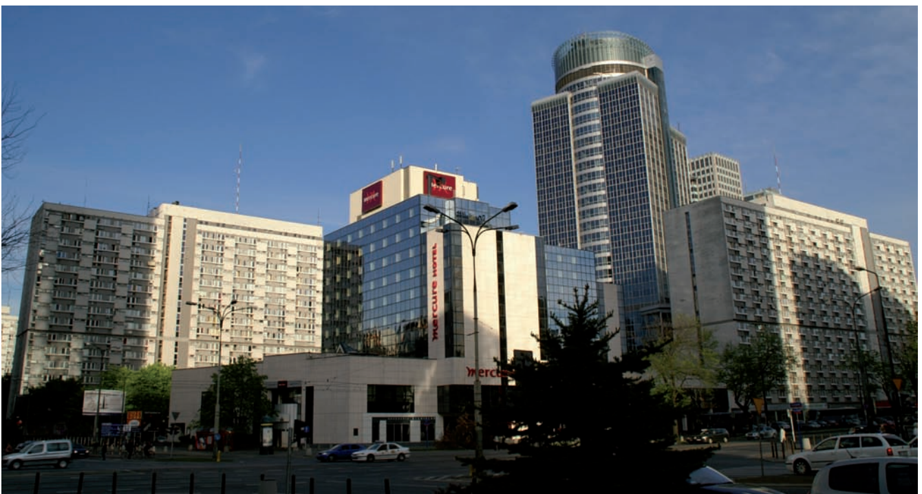
13. Za Żelazną Bramą housing estate in Warsaw, design 1961-65, construction 1965-72. Architects: J. Czyż, J. Furman, J. Józefowicz, A. Skopiński. Current state with hotel and office buildings introduced in between the housing development over the last two decades. Photo by J. Roguska, 2009
