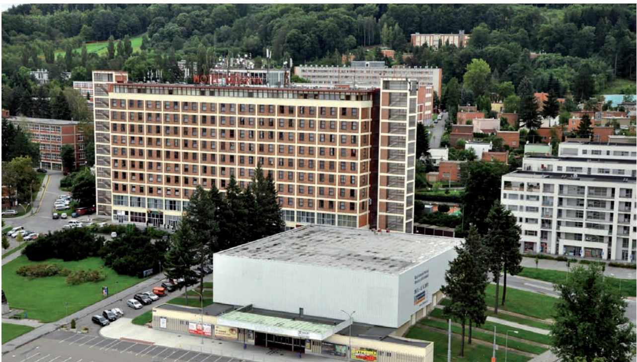
5. Zlín, typical factory building. Photo by A. Syska, 2010
