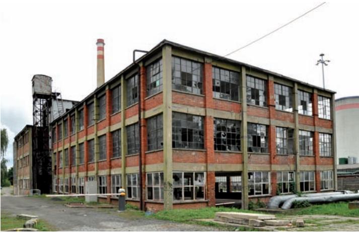
3. Zlín, typical factory building. Photo by A. Syska, 2010
