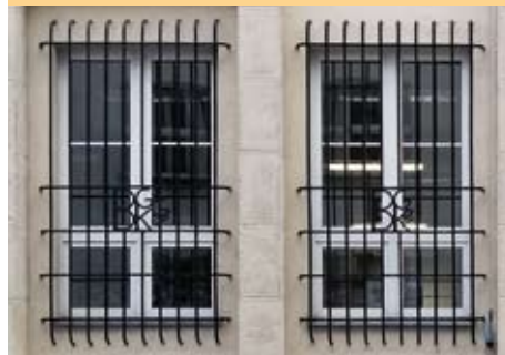
19b. Budynek BGK 19b. BGK building
