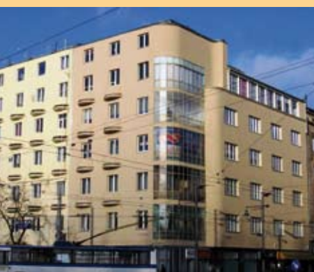
12a. Kamienica 12a. Apartment house
