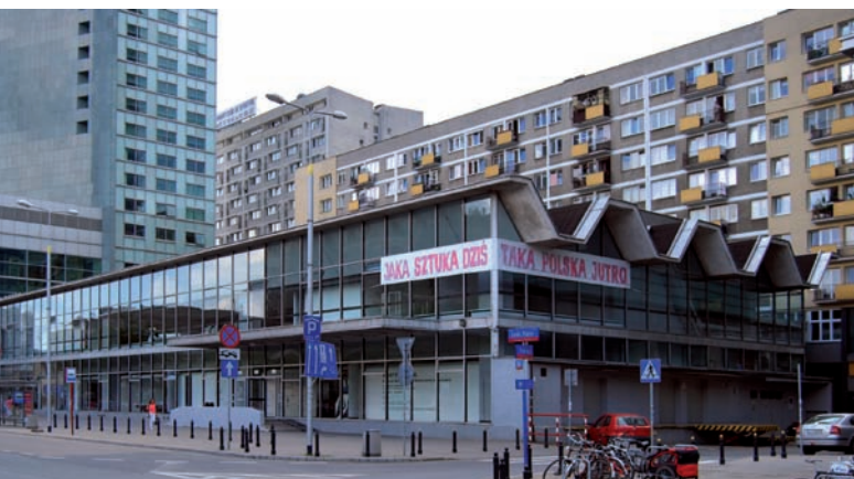
1. Warsaw, pavilion "Emilia", designed by Marian Kuźniar, Czesław Wagner, 1967-69, which was not put on the List of Contemporary Culture Heritage but was entered with procedural errors into the monument register from which it was subsequently removed. Subject of broad discussion concerning the purpose of protecting a modernist building, caused by previous lack of recognition of its value. Photo by J. Lewicki, 2013
