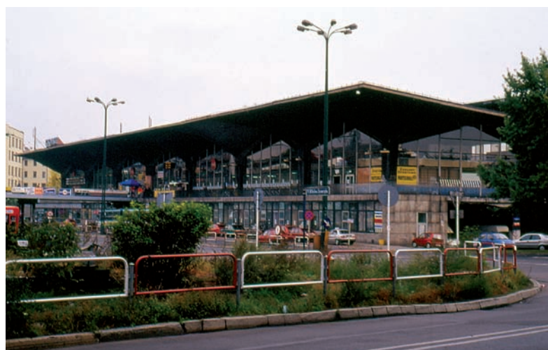
6. Katowice, railway station, designed by Waław Kłyszewski, Jerzy Mokrzyński and Eugeniusz Wierzbicki, 1966-1972. Example of a building of recognised architectonic and aesthetic value, generally regarded as the most precious Polish example of brutalism, which the Silesian Monument Conservator, refused to enter into the heritage register, as a result of which the building was demolished and replaced with a new one. Photo by J. Lewicki, 2007
