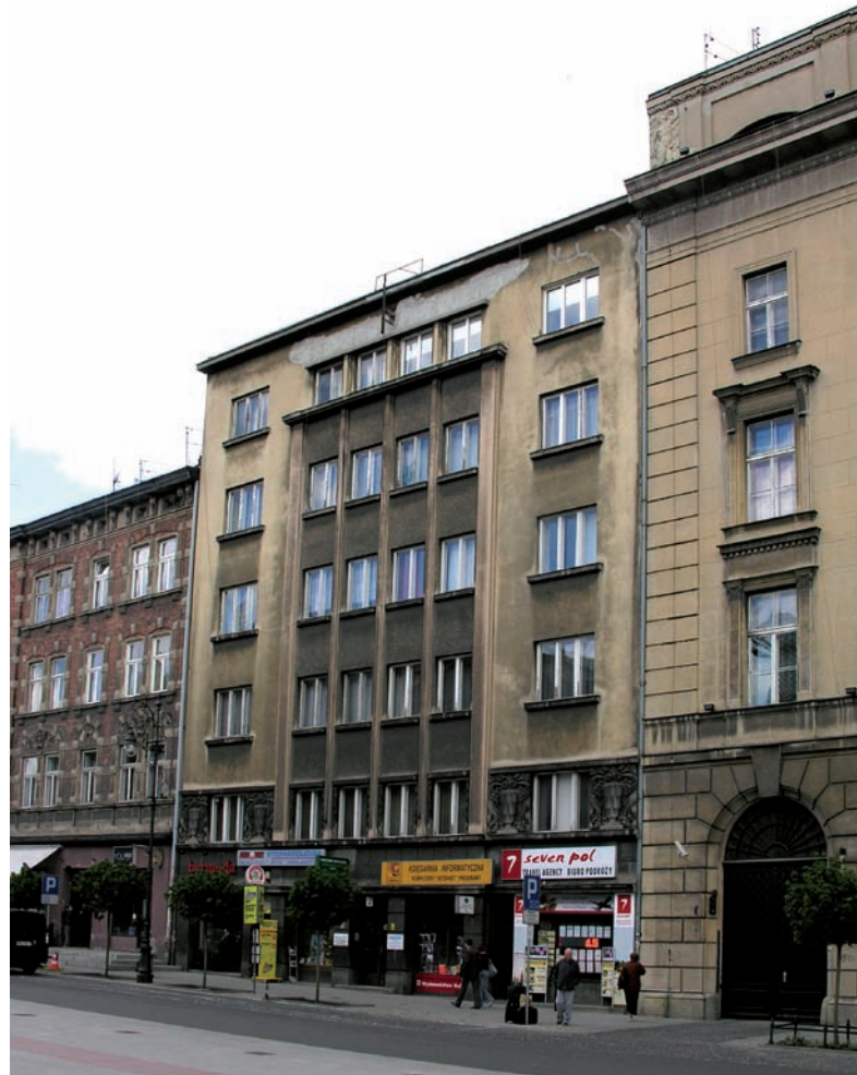
5. Town house in Plac Matejki 2 in Kraków, Fryderyk Tadanier, 1938-40. Photo by B. Makowska
