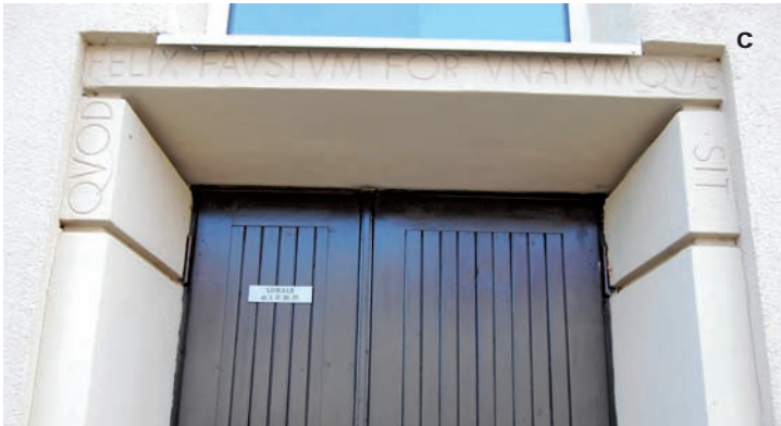
3. Typical elevation of a residential building after insulating it using the dry method. Visible change in the texture, colouring and finishing of the façade. 3a. General view of the building; 3b. Central fragment of the insulated elevation; 3c. Fragment of the entrance – visible “disappearance” of once protruding architectonic frame of the entrance and deformation of the sentence around the entrance. Warsaw, 19 Wawelska St., designed at the beginning of the 1930s. Photo by J. Lewicki, 2010
