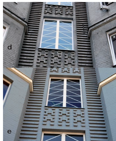
5. Elevation from grey cement brick laid in patterns. State before and after conservation renovation - Warsaw, tenement house belonging to the Spółdzielnia Budowlano-Mieszkaniowa "Grójecka 40A", 40a Grójecka St., designed by Władysław Nałęcz Raczzyński, 1930-31. Visible deformations in texture and colouring resulting from preserving secondary accumulations on the bricks during conservation work, and leaving them as chronologically valuable layers. 5a. General view; 5b-5c. Central fragment of the elevation. State before and after the work; 5d-5e. Detail, view. State before and after the work. Photo by J. Lewicki, 2010
