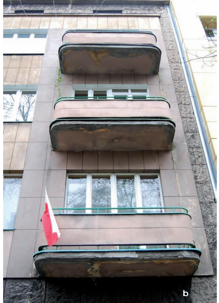
8. Elevation covered with fine plaster, top coat coloured in mass, in the bottom part an addition imitating stone clinker, visible different intensity of colour in the central and side sections of the façade. Łódź, tenement house in Skwerowa St. (now: Polskiej Organizacji Wojskowej 7), designed by the office of "I. Gutman and L. Oli", second half of the 1930s. 8a. General view; 8b. Fragment of elevation. Photo by J. Lewicki, 2010
