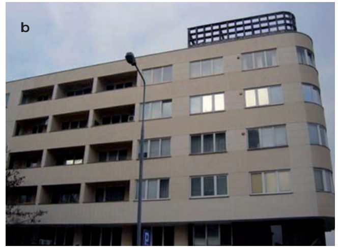
6. Warsaw, Wedel House, 28 Puławska St., designed by Juliusz Żórawski, 1935-38. A model building from the current of luxurious functionalism. Example of elevation destruction as a result of not recognising its high architectonic value. 6a. Façade before the plaster replacement; 6b. View after the plaster replacement. Photo: J. Lewicki 2008-2010. Visible differences in colouring and texture of the new finish. Architect J. Żórawski believed the plaster finish with a uniform finishing coat and variety of colour to be the most important element of the façade finish, which is confirmed by his recorded comments and accounts of workers erecting the building. The ideal finishing coat of the newly applied plaster was controlled by Żurawski at night by means of special lanterns illuminating it from the bottom upwards, which revealed all the irregularities and colour differences
