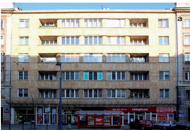
4. Elevation lined with sandstone. Visible discolouration of stone resulting from improper cleaning of the elevation. Warsaw, Oskar Robinson’s tenement house, then of the Związek Emerytów BGK, 18 Marszałkowska St., designed by Lucjan Korngold 1935-36. 4a. General view; 4b. Fragment of elevation. Photo by J. Lewicki, 2009
