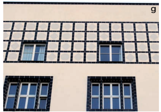
10. Conservation of elevation covered with multi-layer plaster and ceramic clinker facing. Kraków, House of the UJ Professors, the corner of 15 Słowackiego and 61 Łobzowska streets, designed by Ludwik Wojtyczko 1929, realisation until 1932. 10c.-10d. View of side elevation. State before and after the work; 10e.-10g. Fragments of elevation, state after the work. Photo by J. Lewicki, 2007 and 2010
