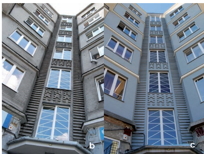
5. Elevation from grey cement brick laid in patterns. State before and after conservation renovation - Warsaw, tenement house belonging to the Spółdzielnia Budowlano-Mieszkaniowa "Grójecka 40A", 40a Grójecka St., designed by Władysław Nałęcz Raczzyński, 1930-31. Visible deformations in texture and colouring resulting from preserving secondary accumulations on the bricks during conservation work, and leaving them as chronologically valuable layers. 5a. General view; 5b-5c. Central fragment of the elevation. State before and after the work; 5d-5e. Detail, view. State before and after the work. Photo by J. Lewicki, 2010
