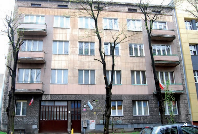
8. Elevation covered with fine plaster, top coat coloured in mass, in the bottom part an addition imitating stone clinker, visible different intensity of colour in the central and side sections of the façade. Łódź, tenement house in Skwerowa St. (now: Polskiej Organizacji Wojskowej 7), designed by the office of "I. Gutman and L. Oli", second half of the 1930s. 8a. General view; 8b. Fragment of elevation. Photo by J. Lewicki, 2010
