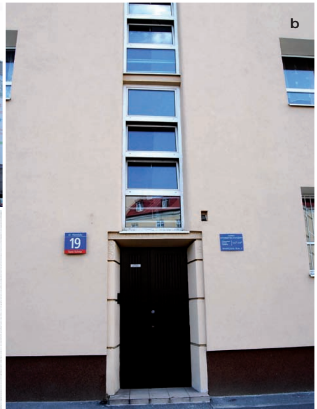
3. Typical elevation of a residential building after insulating it using the dry method. Visible change in the texture, colouring and finishing of the façade. 3a. General view of the building; 3b. Central fragment of the insulated elevation; 3c. Fragment of the entrance – visible “disappearance” of once protruding architectonic frame of the entrance and deformation of the sentence around the entrance. Warsaw, 19 Wawelska St., designed at the beginning of the 1930s. Photo by J. Lewicki, 2010
