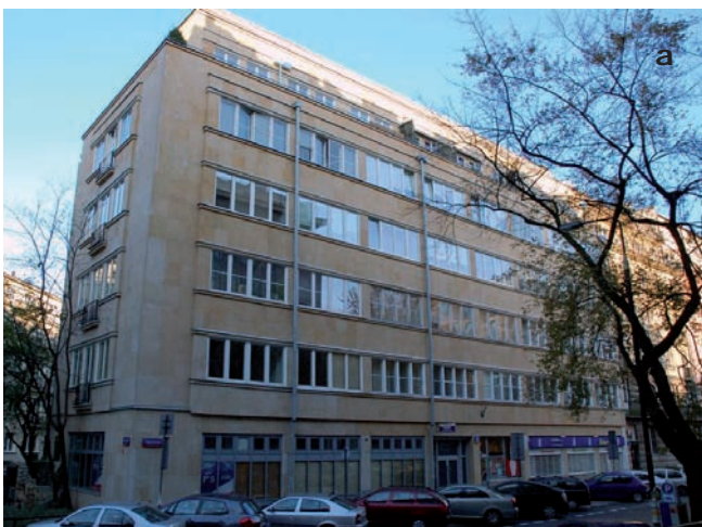
7. Elevation lined with sandstone. Visible slight discoloration, resulting from proper cleaning of the elevation and maintaining it in good condition. Warsaw, O. Robinson's tenement house, corner of 10 Koszykowa St. and Al. Przyjaciół, designed by Lucjan Korngold 1937. 7a. General view; 7b. Fragment of elevation; 7c. Plaque with the architect's name and the original colour scheme re-patinated. Photo by J. Lewicki, 2009
