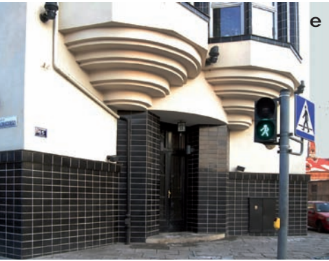
10. Conservation of elevation covered with multi-layer plaster and ceramic clinker facing. Kraków, House of the UJ Professors, the corner of 15 Słowackiego and 61 Łobzowska streets, designed by Ludwik Wojtyczko 1929, realisation until 1932. 10c.-10d. View of side elevation. State before and after the work; 10e.-10g. Fragments of elevation, state after the work. Photo by J. Lewicki, 2007 and 2010
