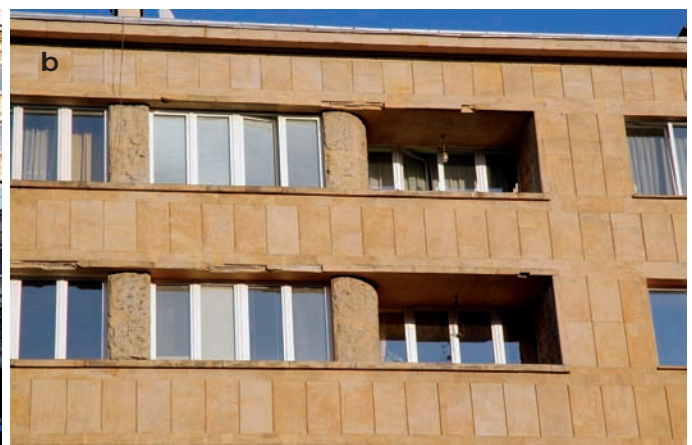
4. Elevation lined with sandstone. Visible discolouration of stone resulting from improper cleaning of the elevation. Warsaw, Oskar Robinson’s tenement house, then of the Związek Emerytów BGK, 18 Marszałkowska St., designed by Lucjan Korngold 1935-36. 4a. General view; 4b. Fragment of elevation. Photo by J. Lewicki, 2009
