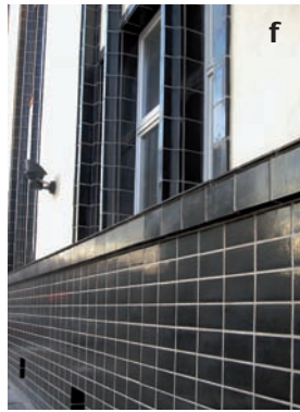
10. Conservation of elevation covered with multi-layer plaster and ceramic clinker facing. Kraków, House of the UJ Professors, the corner of 15 Słowackiego and 61 Łobzowska streets, designed by Ludwik Wojtyczko 1929, realisation until 1932. 10c.-10d. View of side elevation. State before and after the work; 10e.-10g. Fragments of elevation, state after the work. Photo by J. Lewicki, 2007 and 2010
