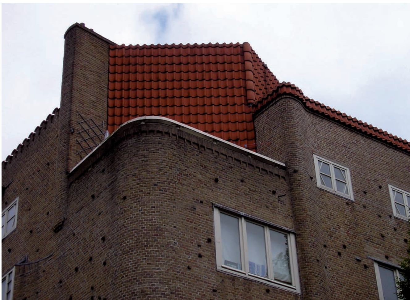
11. An almost dramatic contrast has been developed between the long and rather flat façades opposed to the imaginative plasticity of the corner solutions, where brick and roof tiles are brought into motion in a refined manner
