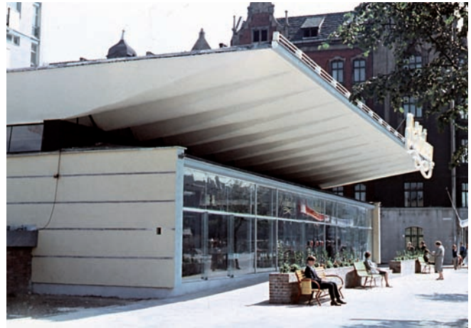
6. Roofing over the entrance to the Delikatesy supermarket. Archive photo from Jurand Jarecki's collection
