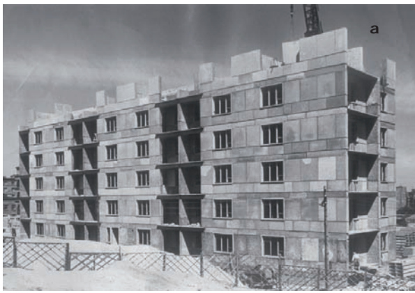
3. A Multi-family residential building at 37, 3 Maja Street, built with grand-block prefabrications in banded arrangement plastered in prefabrication plant: a. the view during construction, b. the current state
