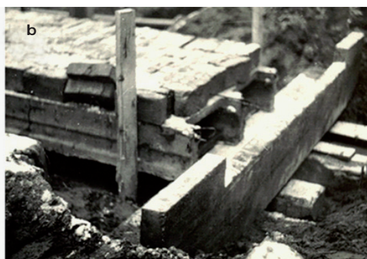
1. Multi-family residential building at 36-44 Abrahama Street built with the use of "modified Leningrad" ceilings: a. the view during construction, b. a detail of the ceiling boards support, c. the walls structural layout with a reinforced concrete half-skeleton prefabricated from H frames with openwork bolt
