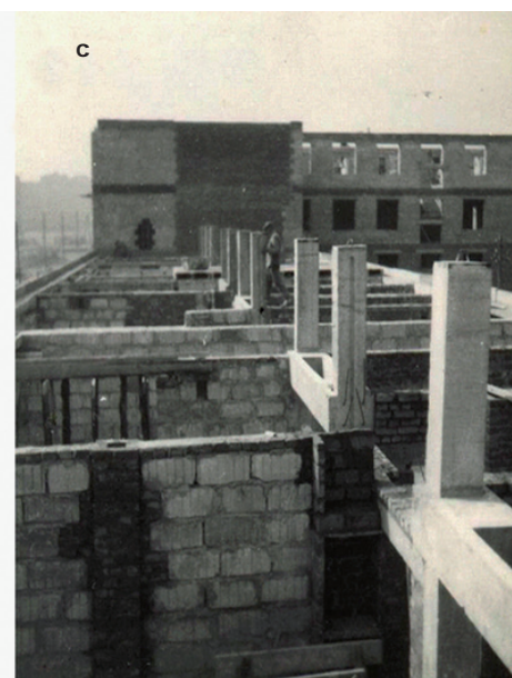
1. Multi-family residential building at 36-44 Abrahama Street built with the use of "modified Leningrad" ceilings: a. the view during construction, b. a detail of the ceiling boards support, c. the walls structural layout with a reinforced concrete half-skeleton prefabricated from H frames with openwork bolt
