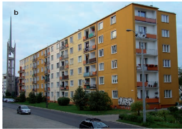
3. A Multi-family residential building at 37, 3 Maja Street, built with grand-block prefabrications in banded arrangement plastered in prefabrication plant: a. the view during construction, b. the current state
