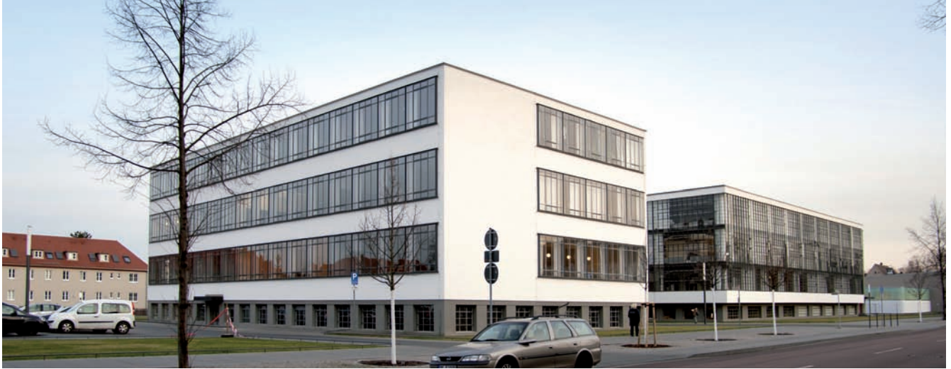
9. North façade of the north wing after the installation of new windows, 2012. Bauhaus Dessau Foundation, Yvonne Tenschert, 2012
