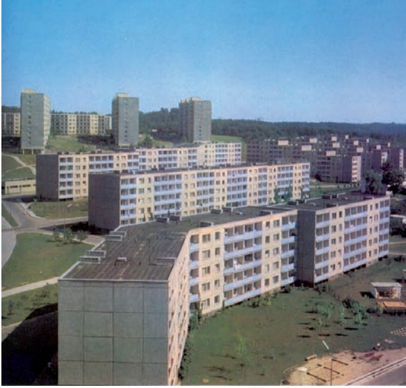
2. A new series of 15 typical apartment buildings, designs for the Lazdynai. The apartment houses were arranged in sections across the relief grade, and of the "broken" plan – along the relief. Photo by M. Sakalauskas in Vilniaus architektūra, Vilnius: Vaga, 1978
