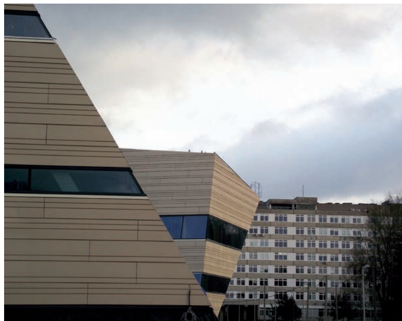
8. The new library (implemented in 2013) by Palekas Arch Studio and modernist volumes Vilnius University, Arch. Rimantas Dičius, Julius Jurgelionis, 1971–75. Photo by L. Nekrošius, 2011
