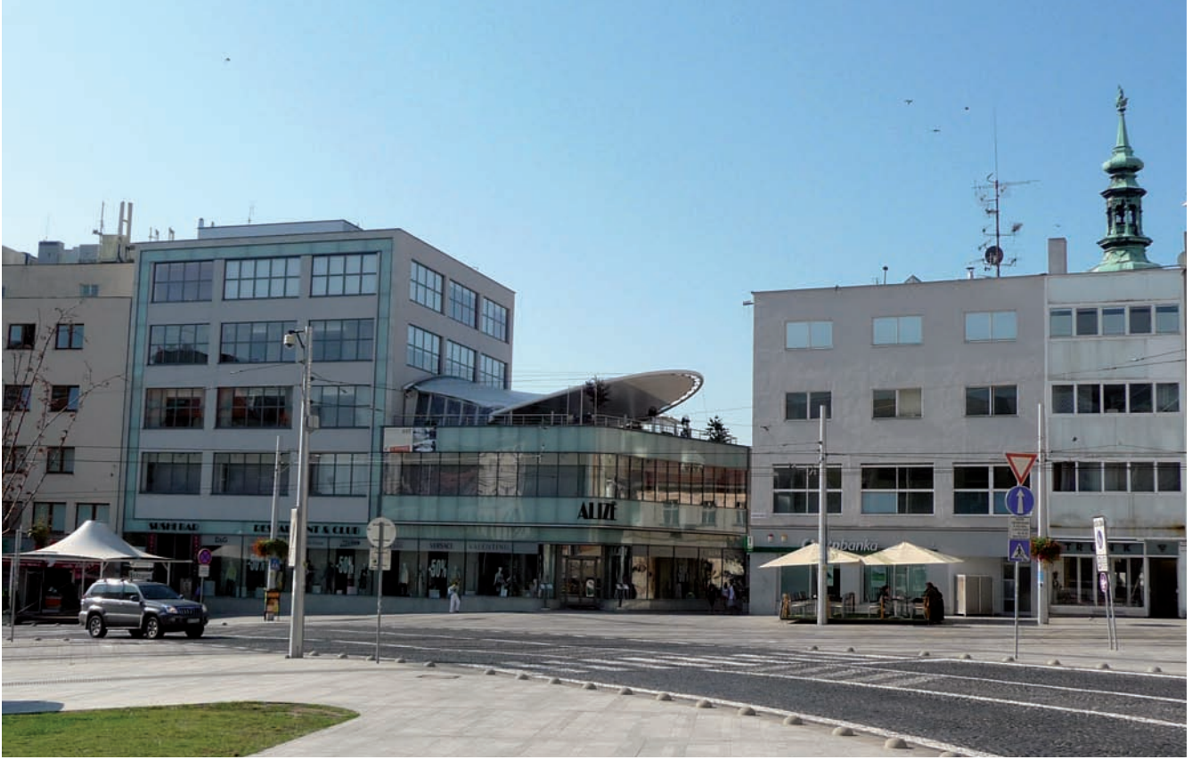
1. Present view of the Baťa Department Store, 1929-31 by Vladimír Karfík. Photo by V. Kapišinská, D. Haberland
