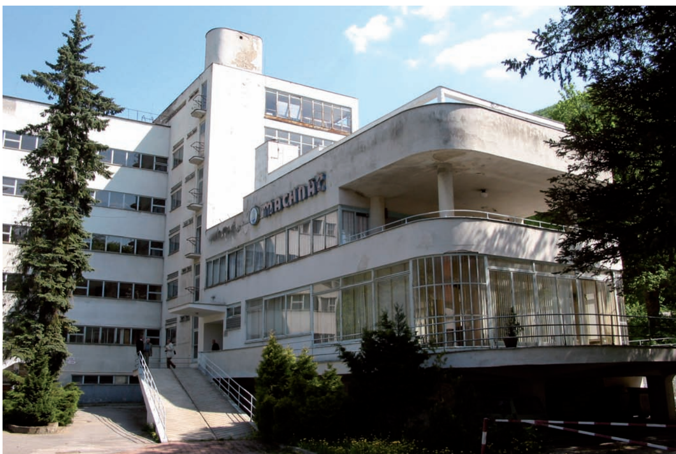
10. Sanatorium Machnáč in Trenčianske Teplice, 1930-32 by Jaromír Krejcar, waiting for reconstruction. Photo by V. Kapišinská, D. Haberland
