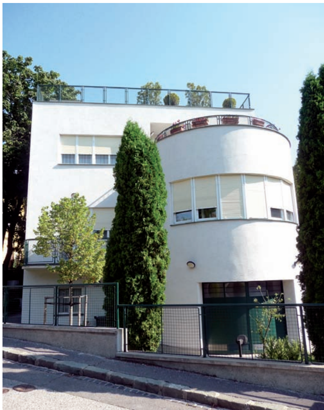
9. Present view of the Villa on Porubského Street 1, 1936-37 by Ernst Spitzer. Photo by V. Kapišinská, D. Haberland
