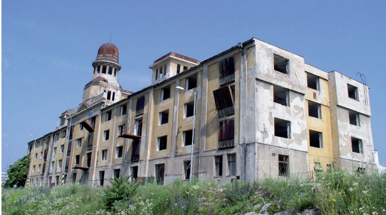
7. View of the abandoned Storage House No. 7 before restoration, 1921-22 by Karol Skorkovský
