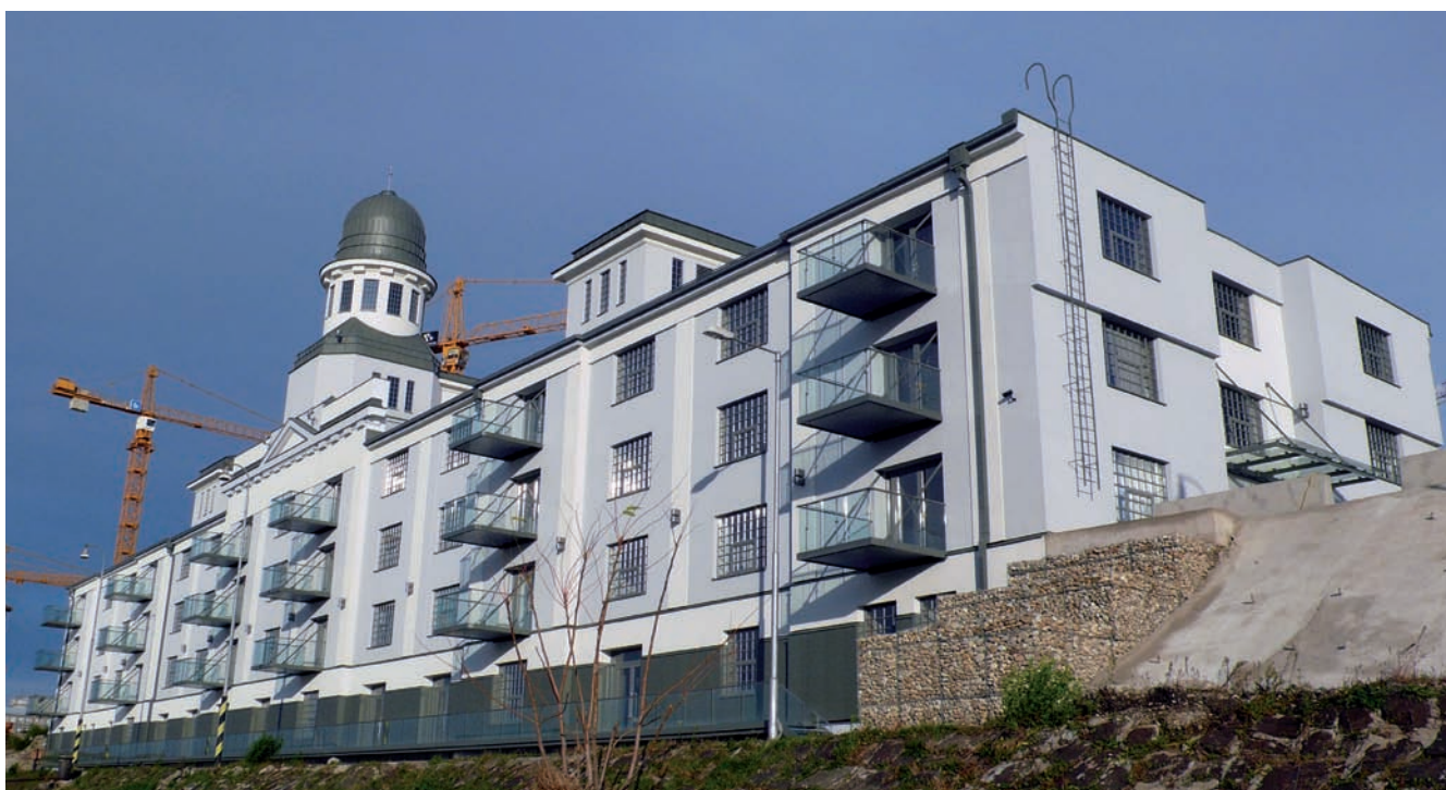
8. Present view of the Storage House No. 7 after restoration in 2006-07. Photo by V. Kapišinská, D. Haberland
