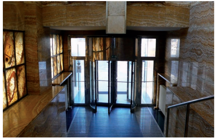
4. View of the staircase entrance facing of onyx of the Slovak Savings Bank. Photo by V. Kapišinská, D. Haberland
