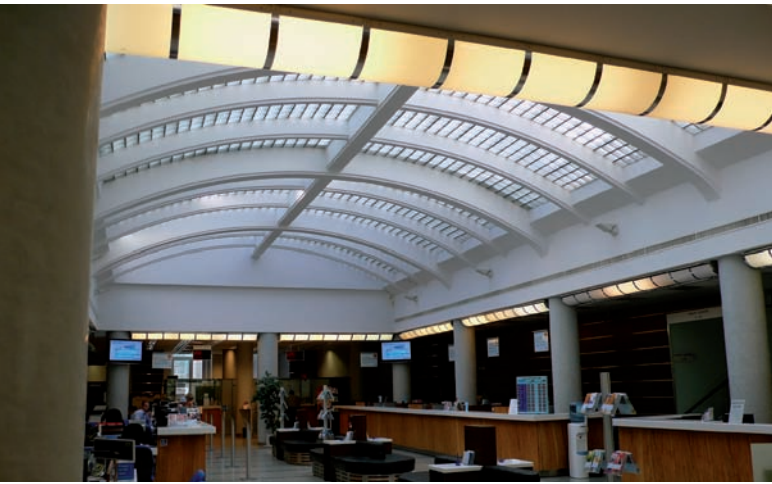
3. Teller hall in Slovak Savings Bank vaulted by glass-concrete arc. Photo by V. Kapišinská, D. Haberland
