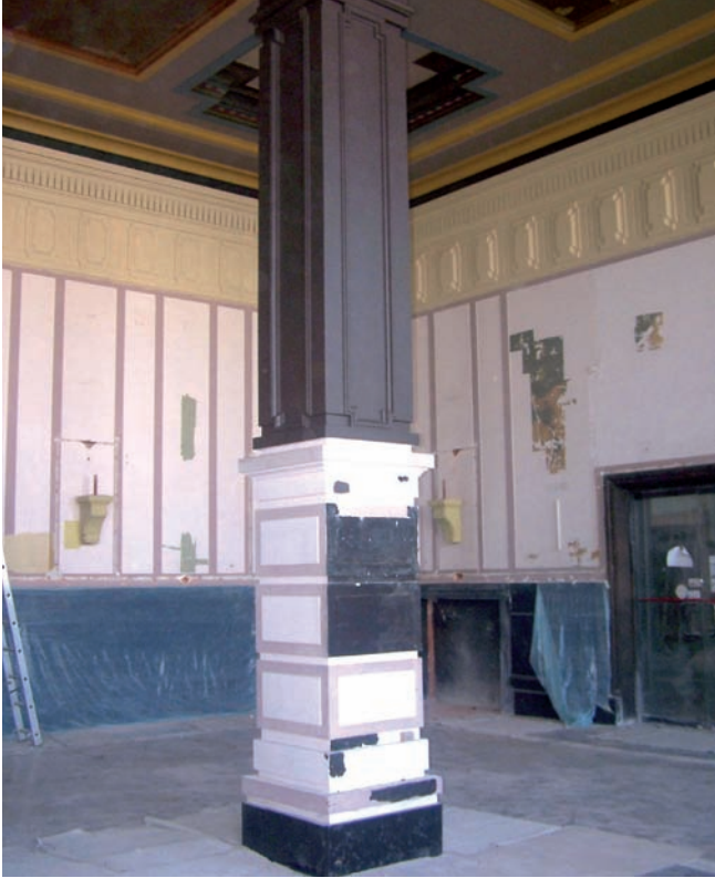
2. Exposed samples of the wooden facing and a colouring test on a column in the restaurant. Photo by A. Kriegseisen
