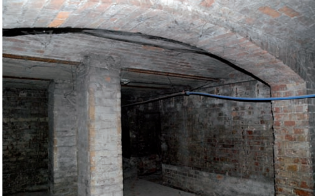
8. Fragment of the old railway station basement, after uncovering. Photo by A. Kriegseisen
