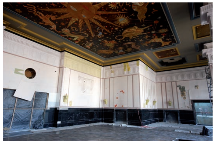
1. Restaurant interior prior to restoration, exposed samples. Photo by A. Kriegseisen
