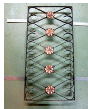
10. Vent grille on the hall ceiling, after restoration. Photo by A. Kriegseisen
