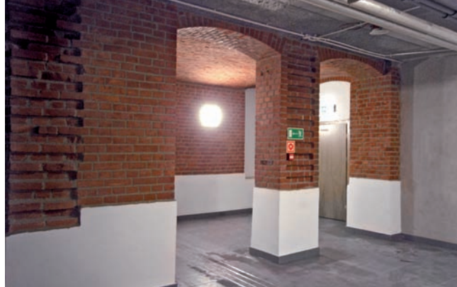
9. Fragment of the old railway station basement, after restoration. Photo by A. Kriegseisen
