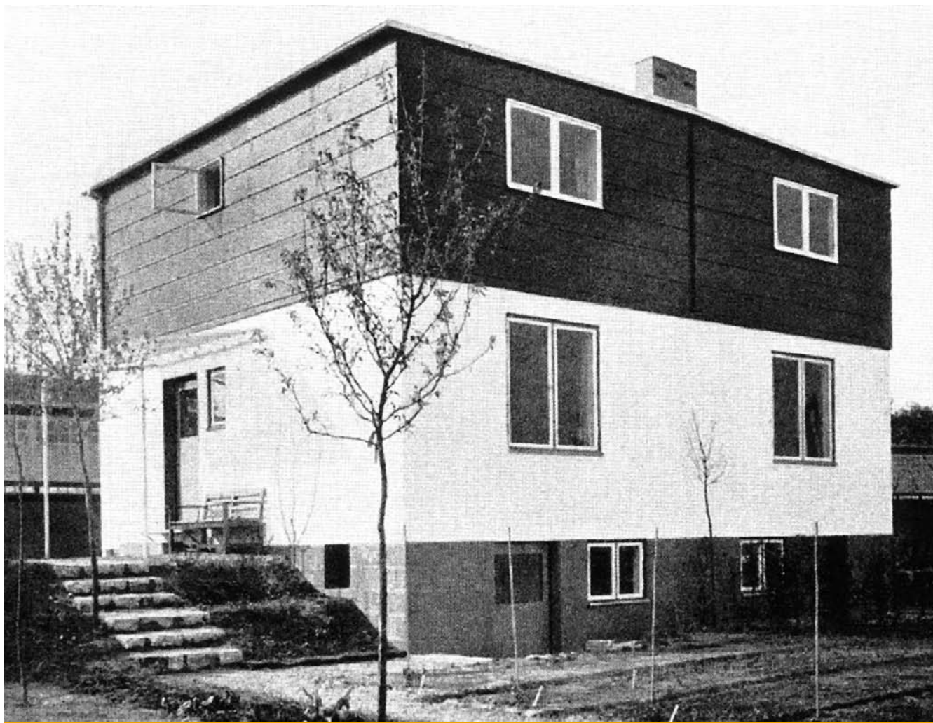
7. "The growing Houses", arch. Egon Eiermann, Fritz Jaenecke and Paul Mebes, Emmerich (source: M. Wagner, Das Wachsende Haus... , op. cit., p. 111 i 83)
