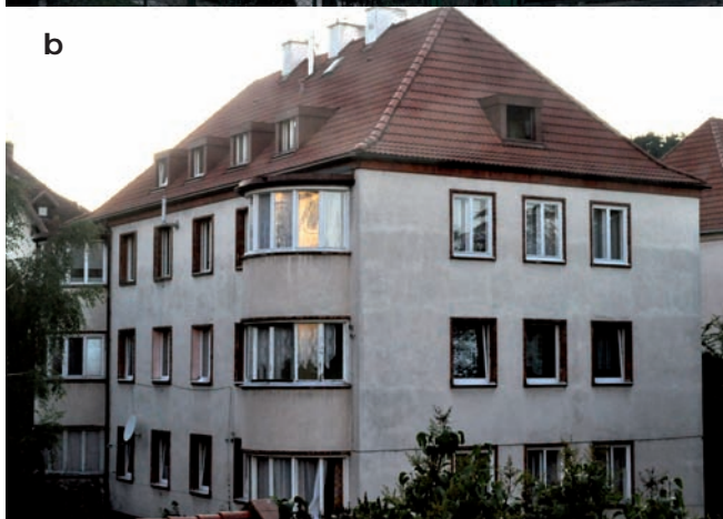
2. Multi-family house, Krótka 1, Sopot, probably designed by Adolf Bielefeldt, ca. 1932: a. frontal façade; b. rear façade. Photo by A. Narczewska
