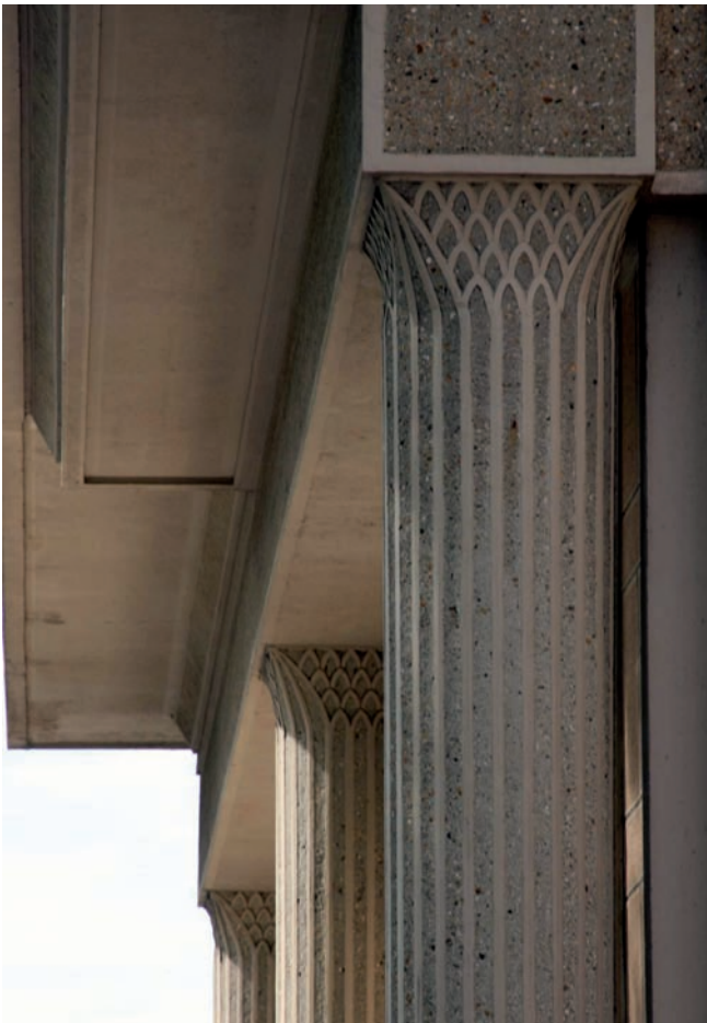
8. A concrete column of the S29 quarter, an illustration of the notion of structural classicism defined by the architect and historian Joseph Abram. © The City of Le Havre
