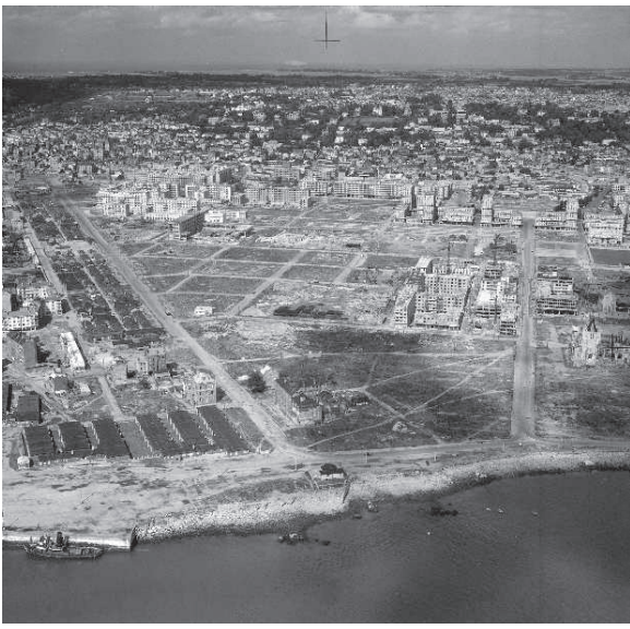
2. View of the city centre during reconstruction, around 1959. © GPMH
