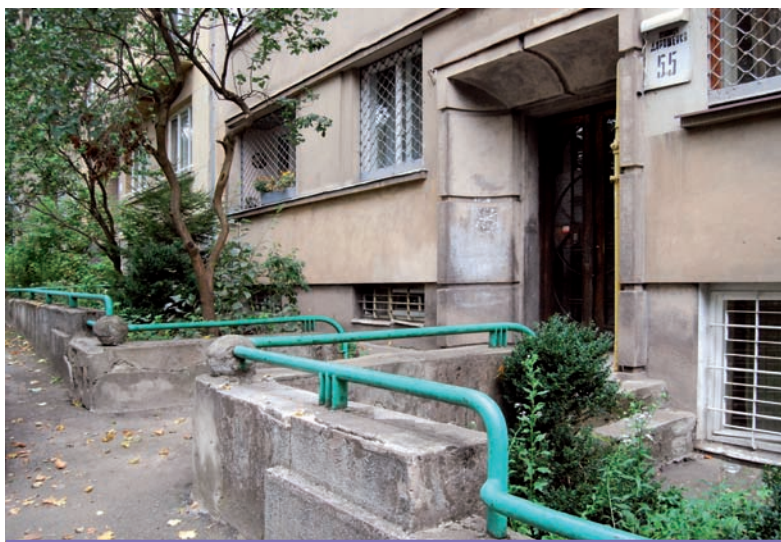
7. Lviv, tenement houses at 49-55 Sykstuska St., now Doroszenki St., design. Salomon Keil and Henryk Sandig, 1937-1938. View of the front garden with preserved modernist walls and banisters (photo M. Korpała)
