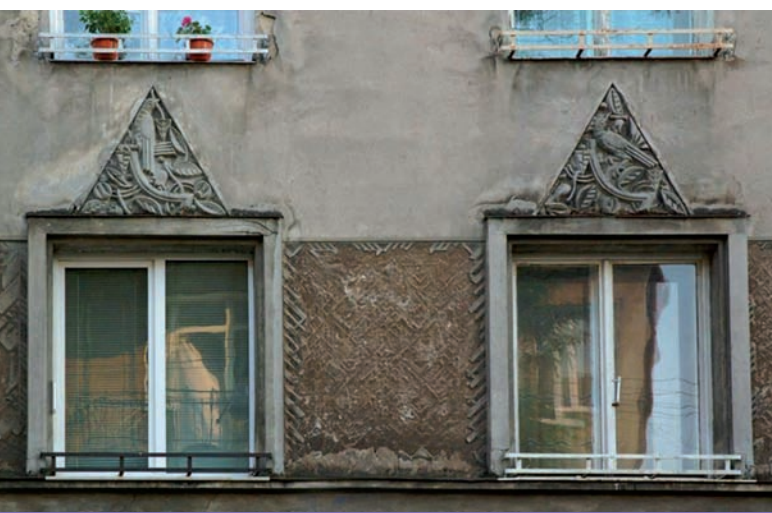
5. Lviv, fragment of elevation of tenement house at 32 Św. Jacka St. (now Archipenki), design. Tadeusz Wróbel, 1929-1931. Sgraffito decoration around windows (photo M. Korpała)
