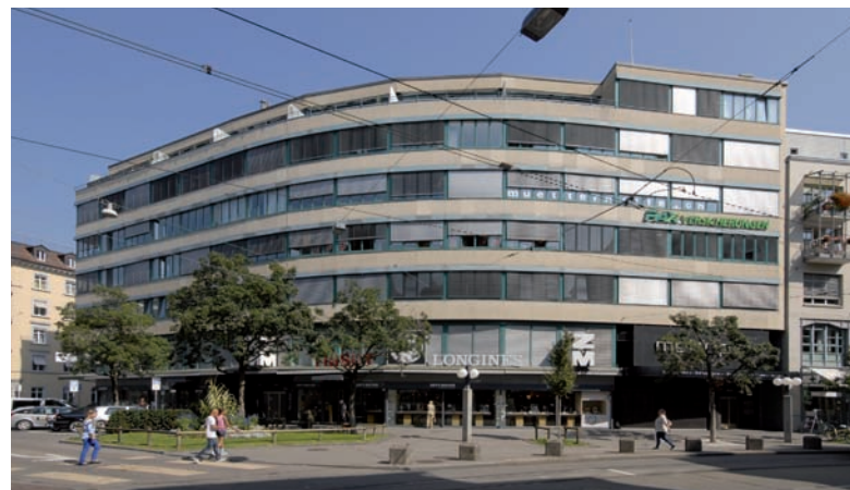
7. The Zed House as it is today. Photo by Werner Huber
