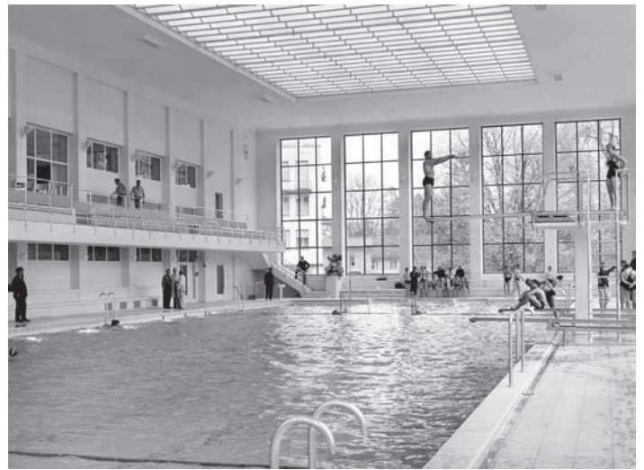
6. The City Indoor Pool, built in 1938–1941. Baugeschichtliches Archiv Zürich, BAZ
