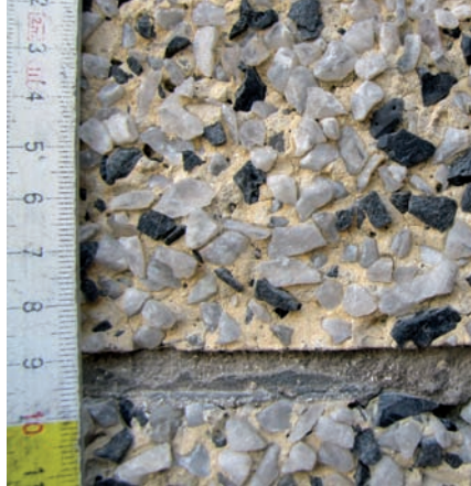
9. A view of the washed render texture on the façade of a townhouse at Świętojańska 47, Gdynia
