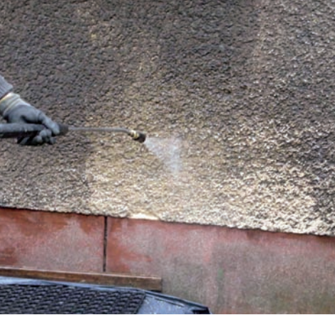
8. The original colour of the 1930s scratch render is revealed during a cleaning procedure (building at Bema 5, Gdynia, 2013)
