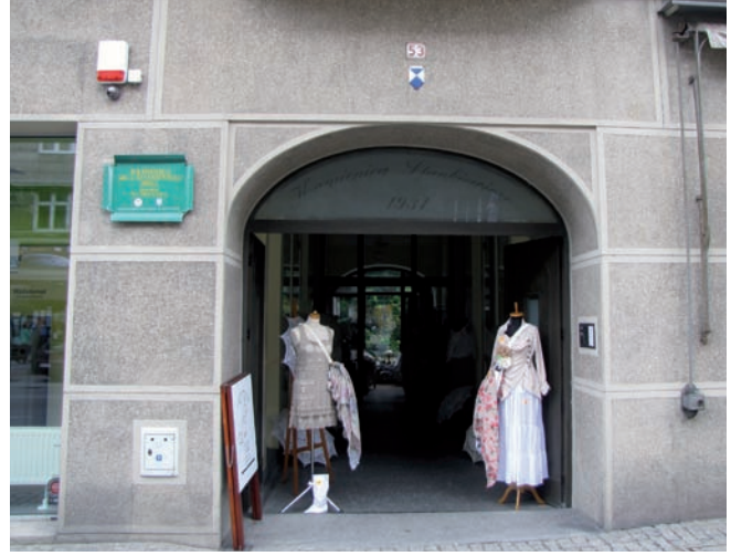
16. Faux stonework finish on the townhouse at Świętojańska 53, Gdynia, stylised to resemble stone cladding
