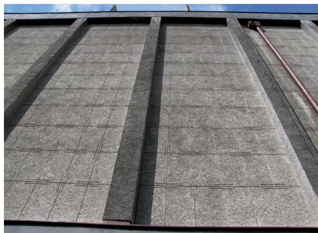
7. Scratch finish applied after World War II on the façade of the Most Sacred Heart of Jesus Catholic Church at Armii Krajowej St., Gdynia
