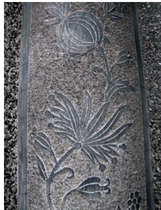
19. Detail of the townhouse portal ornamentation at Wolności 5, Gdynia, with a faux stonework finish folk motif
