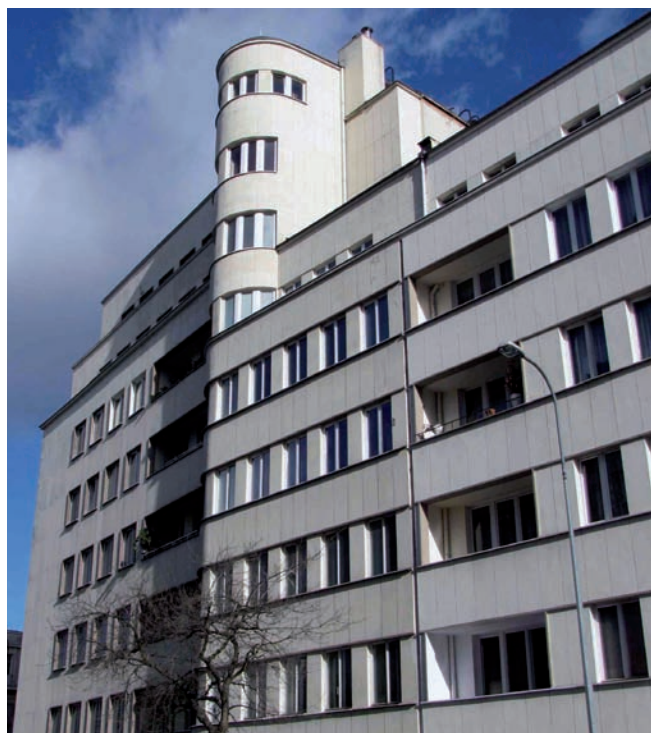
11. Building at 3 Maja 27-31; the façades are finished with natural stone (left-hand side up to the loggias) and imitation stone cladding render (right-hand side with the loggias)
