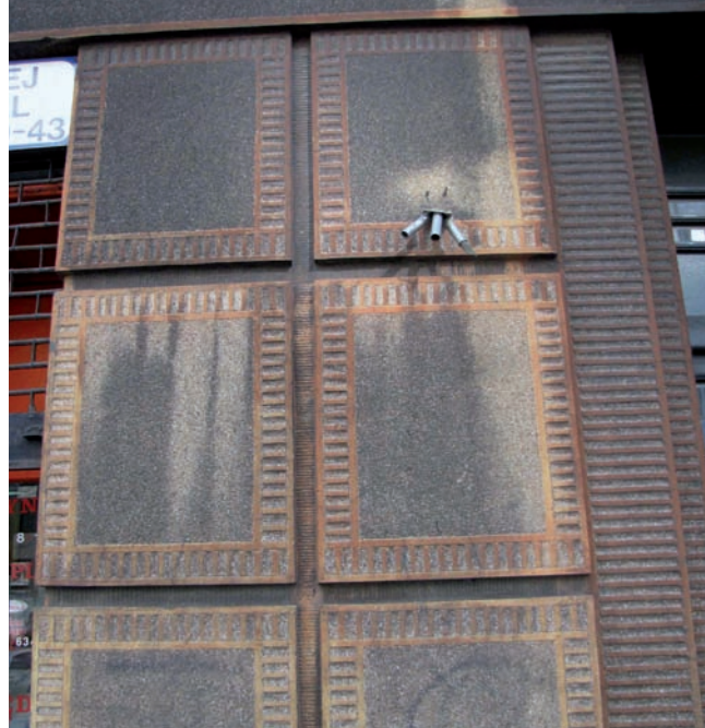
21. Detail of the townhouse façade at Mazowiecka 26a, Kraków, with faux stonework finish
