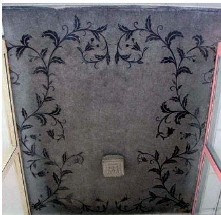
18. Detail of the townhouse ornamentation at Starowiejska 21, Gdynia, with a faux stonework finish folk motif
