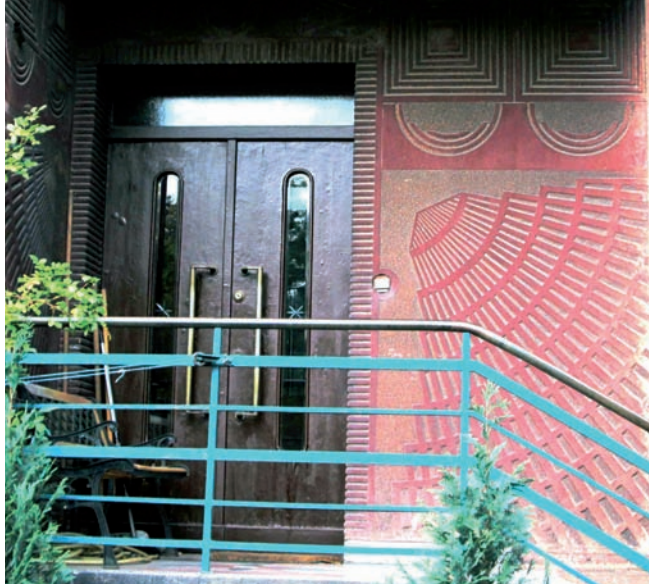
20. Faux stonework finish decoration at the building entrance, at Młyńska 23, Gdynia
