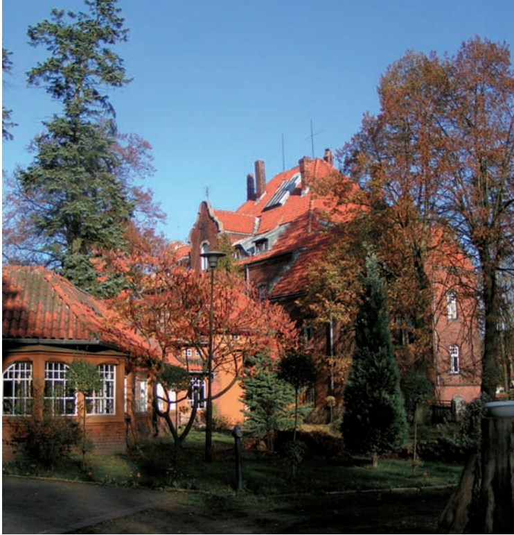
2. Doctor's House joined with sanatorium building by means of a catwalk at the ground level. Photo by B. Bielinis-Kopec
