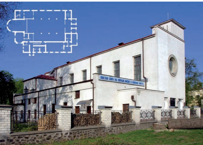
6. Rivne. Sts. Peter and Paul Church, arch. W. Czeczott 1938. View from the East. Measuring by P. Rychkov & O. Mykhaylyshyn. Photo by P. Rychkov, 2009
