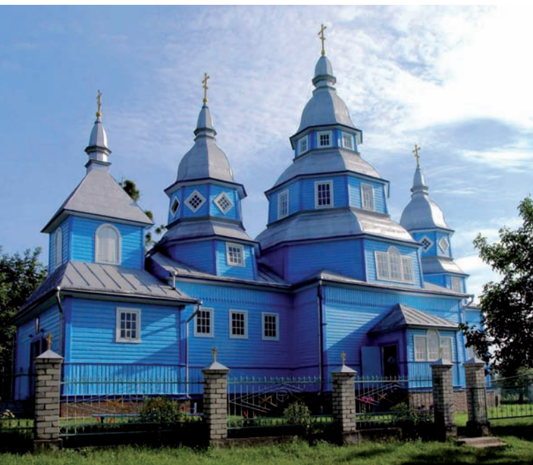
9. Bronniki (village near Rivne). The Mother of God Church, arch. S. Tymoshenko, 1928. Photo by P. Rychkov, 2009
