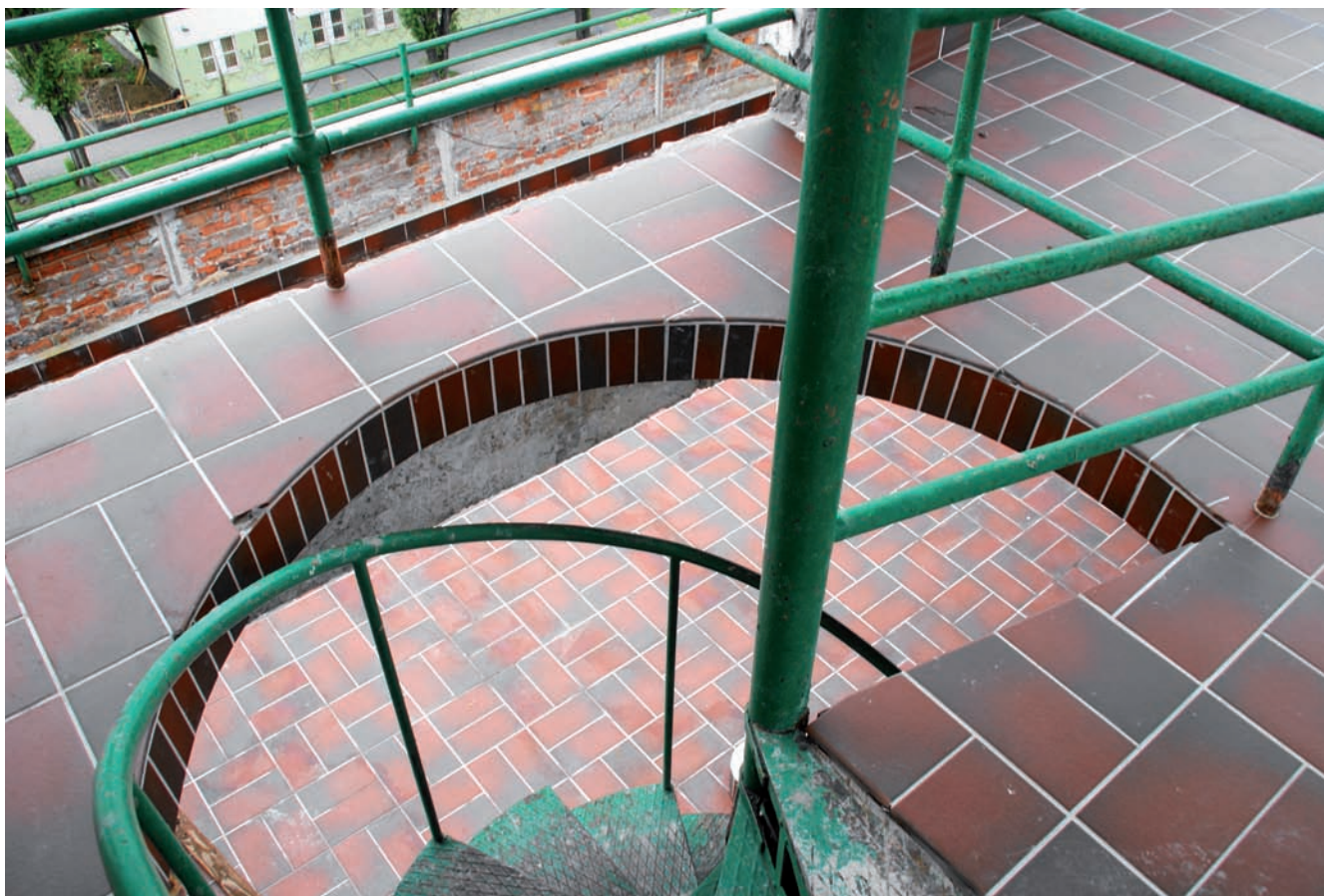
9. Refurbished terrace stairs. Photo by Irena and Andrzej Olszewski
