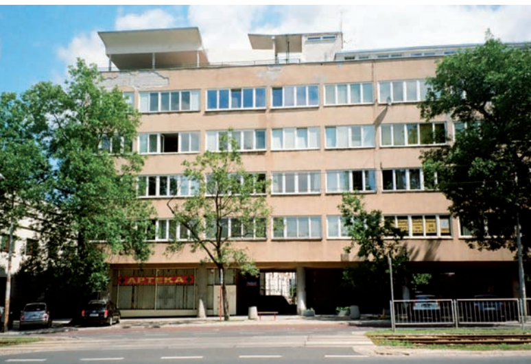
2. The Glass House, view from Mickiewicz Street. Photo by Irena and Andrzej Olszewski
