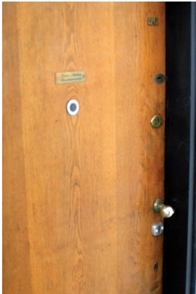
7. Refurbished door. Photo by Irena and Andrzej Olszewski
