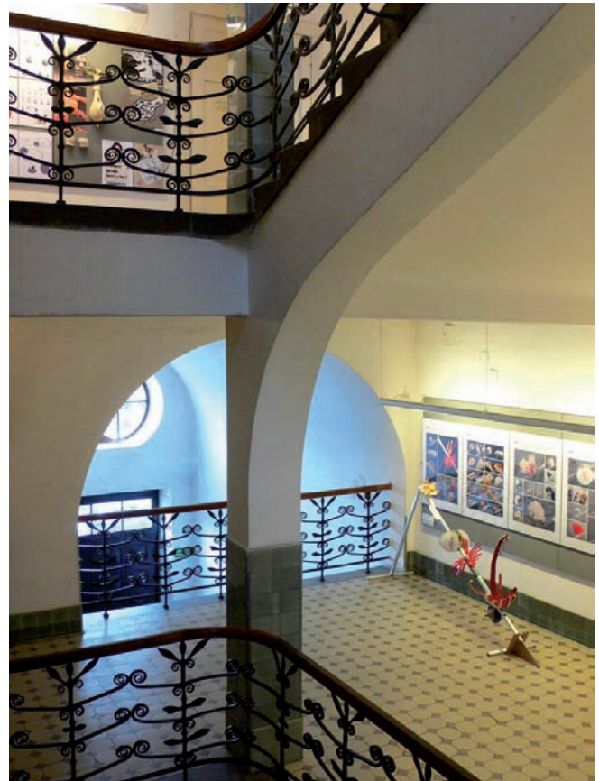
3. Kraków, Academy of Fine Arts Faculty of Industrial Design: the main staircase; ferroconcrete pillar supporting the landing and "softly" transformed into a diagonal beam supporting a flight of stairs. Photo by W. Affelt
