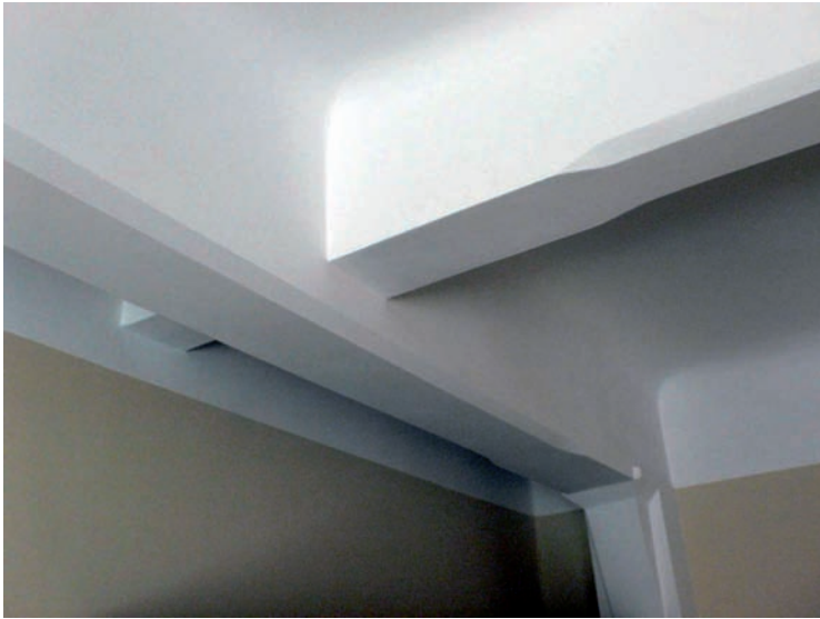
6. Kraków, Academy of Fine Arts Faculty of Industrial Design: detail of the massive ferroconcrete floor structure; what draws attention here is the shape of the edge of the ferroconcrete elements mimicking traditional carpentry woodwork. Photo by W. Affelt
