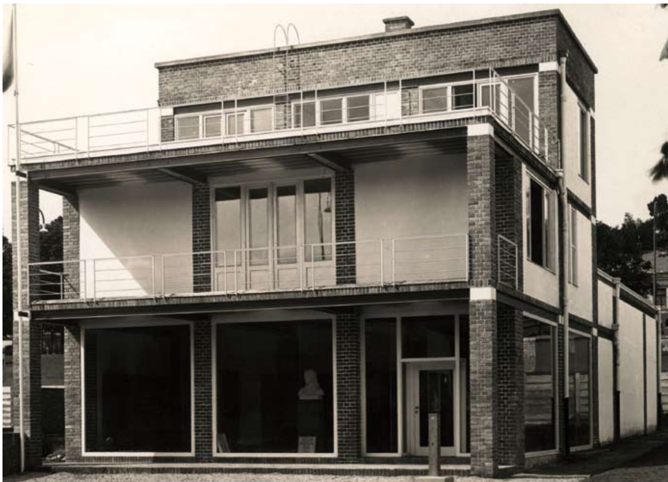
14. Brno, fair grounds, pavilion of the Industrial Art School Prague, Pavel Janák, 1928; pillars consisting of visible brick displayed in module system: two long sides + perpend and three small sides + two perpend; horizontal T-bars painted gray; the walls and the impost zone of the pillars are accented with yellowish-white whitewash on a grated brownish-yellow plaster, that is pigmented with fine sand, very similar to the facade of the Tugendhat House (photo: courtesy NTM Prague, 1928)
