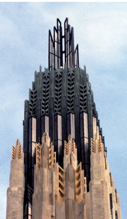
7. The Boston Avenue Methodist Church, Tulsa; tower detail
