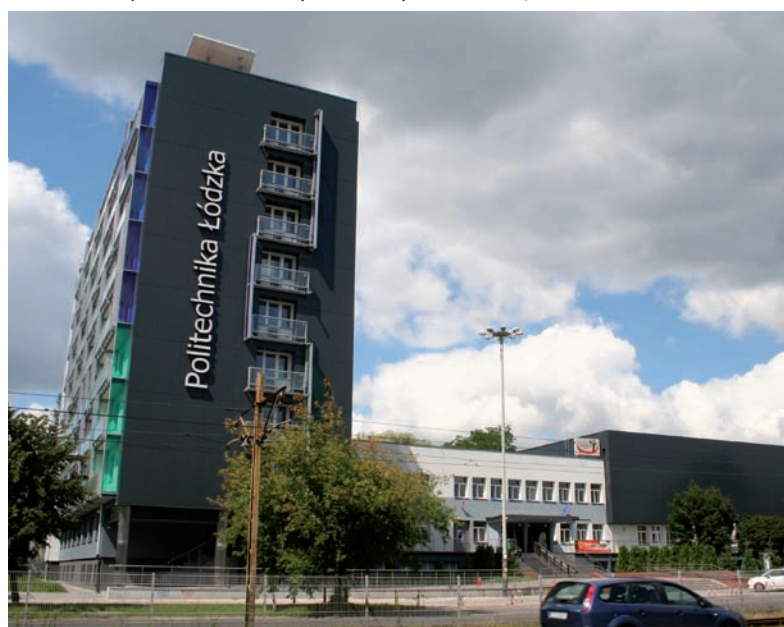
4. Technical University of Łódź building complex (dorm, canteen and cinema performance hall). Photo by the author, 2012
