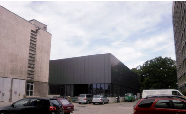
6. Civil Engineering Faculty and the Architecture Department, Technical University in Łódź. Photo by the author, 2012
