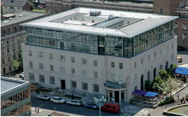
8. Curtis Green RA, Son & Lloyd: Barclays Bank, Plymouth (1949-52). Listed Grade II. Roof additions and alterations, 2006
