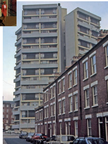
10. Denys Lasdun: Keeling House, Bethnal Green London (1957-59). Listed Grade II* in 1993. Converted to luxury flats in 1999
