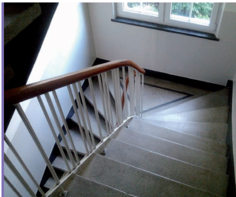
3. I. Goldberger 1937, staircase in the so-called „triangular” style. Terrazo cladding has sustained intact. (Author's photo, 2017)
