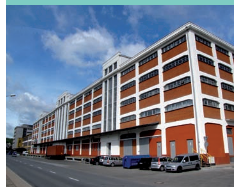
36. Long Term Storage Facility H, Polska 17 St. - after restoration
