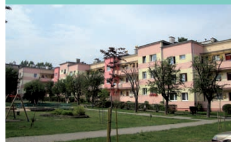
7. Houses of Gdynia Housing Cooperative, Okrzei 2/4 St.
