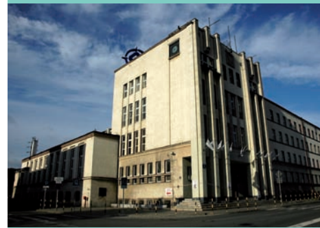
25. Gdynia Port Authority building, Rotterdamska 9 St.
