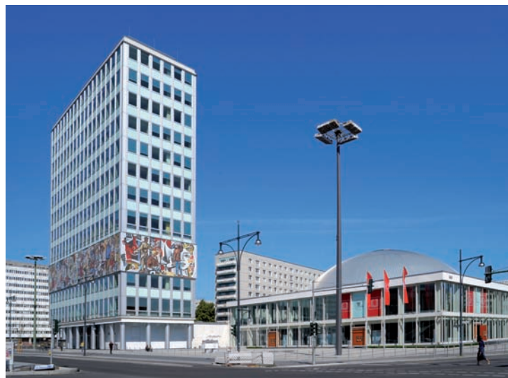
12. The Congress Hall Alexanderplatz (today Berlin Congress Center – BCC) and the "House of the Teacher" in Berlin-East (by Hermann Henselmann, 1961-64): marking the end of the second construction stage of the Karl Marx Avenue. Landesdenkmalamt Berlin / Wolfgang Bittner
