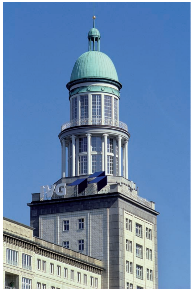
5. Karl-Marx-Allee, first construction stage – the domed tower at Frankfurter Tor is a citing the towers the baroque classicist towers of the French and German cathedral at Berlin Gendarmenmarkt. Landesdenkmalamt Berlin / Wolfgang Bittner
