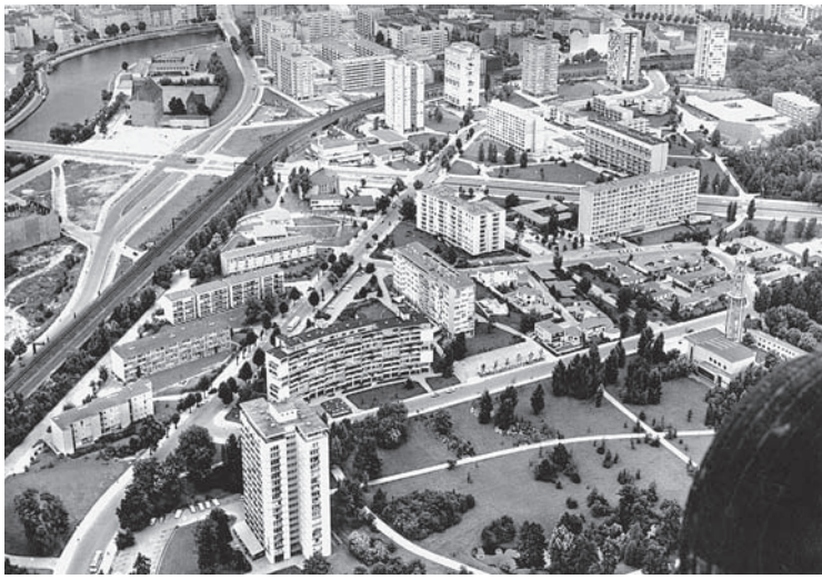
6. Aerial photograph of the Hansa District (Hansaviertel) and the International Building Exhibition 1957 (Interbau '57). Landesdenkmalamt Berlin / Archive
