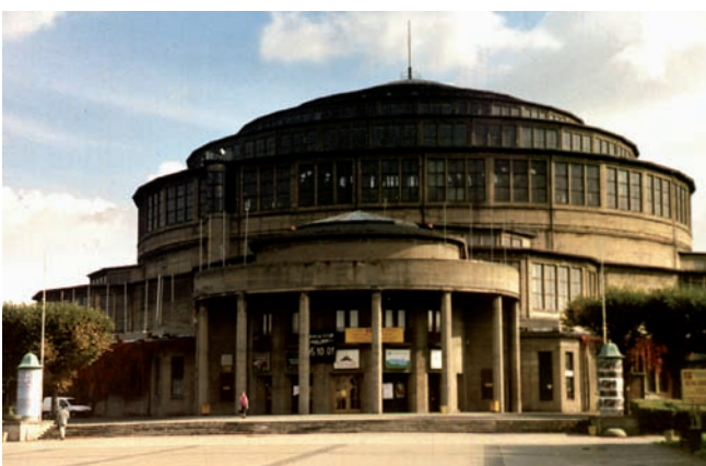
11. Centennial Hall – Hala Ludowa Wrocław (1911-13) by Max Berg, an early modern heritage site in Poland, inscribed on the World Heritage List in 2006. http://commons.wikimedia.org/wiki/File:Wroclaw_hala_ludowa6.jpg / shaqspeare 2001, scanned 2005
