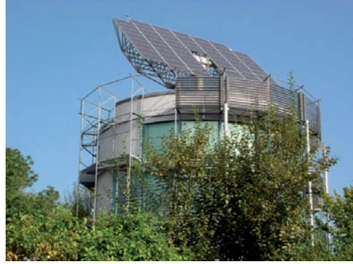
4. The Solar House "Heliotope", Freiburg designed by R. Disch. Photo by the author
