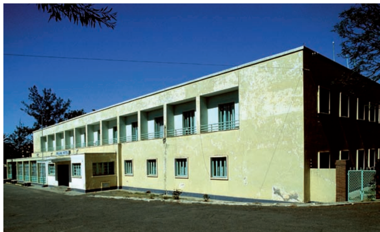
4. The Selam Hotel (1937), designed by Rinaldo Borgnino. Photo by the author
