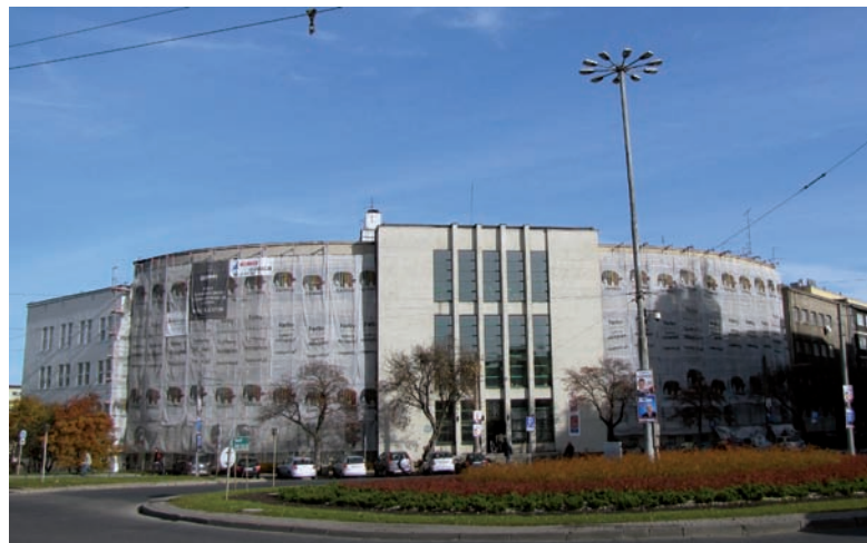
8. Façade conservation of the historical Court of Justice, 2010. Photo by R. Hirsch
