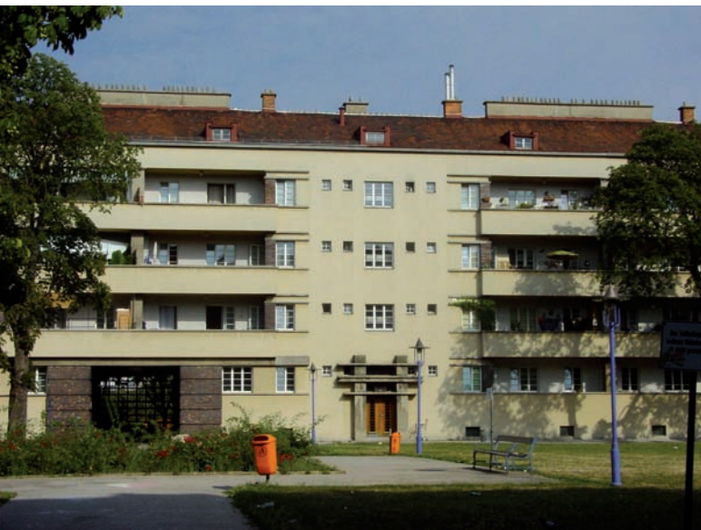
3. The yard in Karl-Marx-Hof housing estate in Vienna. Photo by the author
