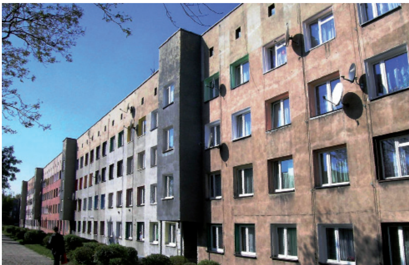
5. Gallery-access building in Roosevelta street ; stripes of avant-garde oriel windows, partly walled up in the 1960s, can be seen. Photo by the author, 2007
