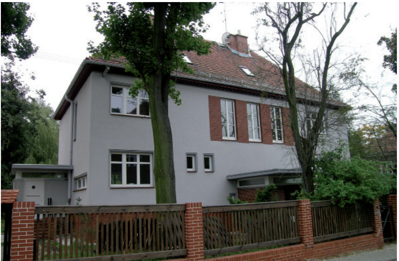
3. A modernised building in the 1920s estate in Ligonja street, Gliwice. Evidently, a lot of effort was put to harmonise new elements with the original style. New windows and fence segments copy their original forms, roof tiles are original, the porch matches the style of the building. This is an example of a growing tendency to recognise the 1920s and 1930s architecture as valuable. The original form and detail are more respected now, which can be noticed in many refurbished houses. Photo by the author, 2007
