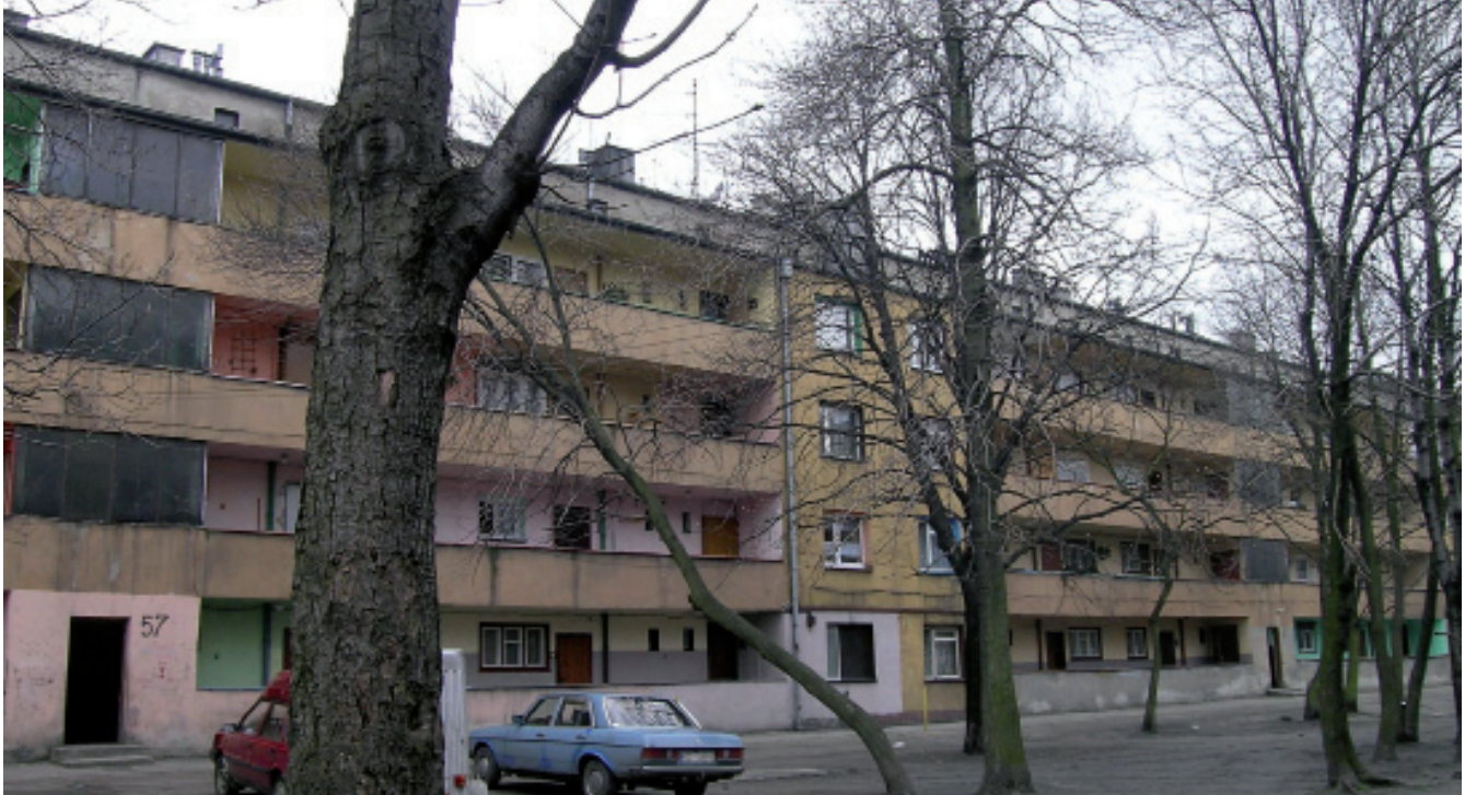
6. Gallery-access building, back view. At present, the building is administered by a number of communities. Each are planning heat insulation on their own, therefore the façade will lose its homogeneity. Photo by the author, 2005
