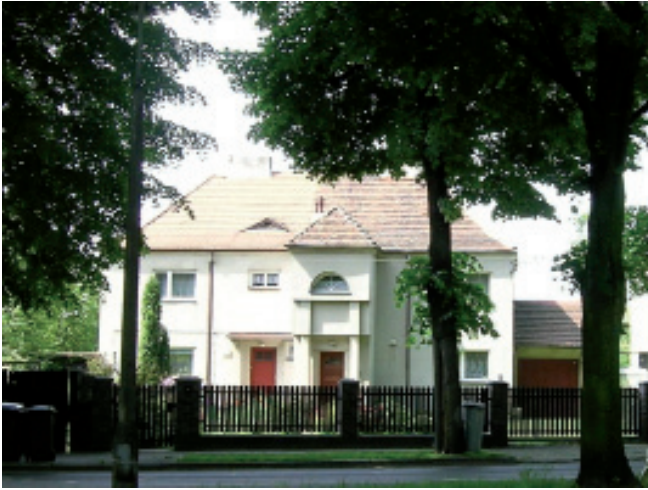
2. Post-Modernist remodelling (1992) of a building in the 1920s estate in Mickiewicza street, Gliwice. Photo by the author, 2008
