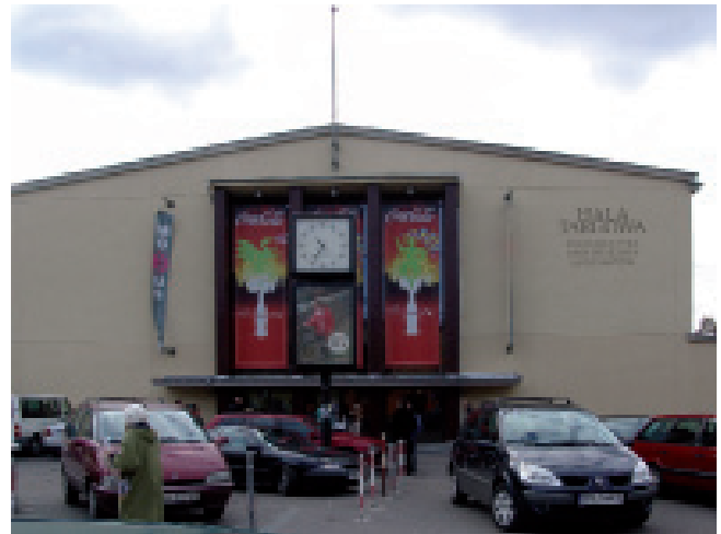
5. Cracow, Covered Market at 3, Daszyńskiego, Juliusz Dumnicki, 1939. Entrance. Photo by the author
