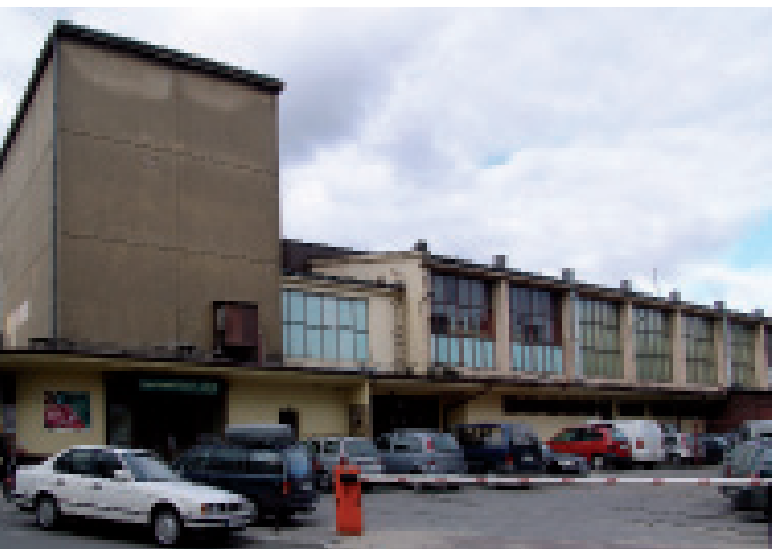
7. Cracow, Covered Market at 3, Daszyńskiego, Juliusz Dumnicki, 1939. Rear view. Photo by the author
