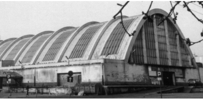
10. J. Müller, S. Reychman, Covered market in Gdynia, 1935-1937. Photo: Archives of Contemporary Architecture, Design Theory and Methodology Department, Faculty of Civil Engineering and Architecture of Szczecin University of Technology
