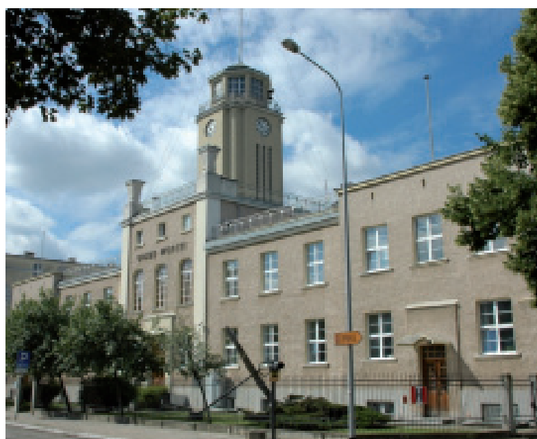
2. Gdynia, Maritime Office at 10, Chrzanowskiego, architect Adam Ballenstedt, 1927. Photo by Maria J. Sołtysik
