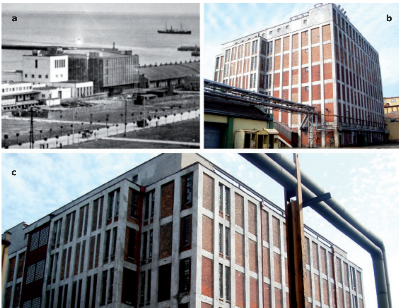
4. Herring Cold Store, Nabrzeże Angielskie, constructed in 1935-36 (Stage 1) and 1960-65 (Stage 2); a. the 1930 archive photograph (from Gdynia Museum collection); b. view on Cold Store from the wharf; c. a grid of reinforced-concrete framing filled with brickwork – fragment of side wall of the Cold Store. Contemporary photographs by A. Orchowska-Smolińska
