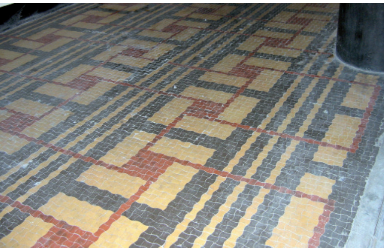
5. Small-tile flooring in the doorway of former FE BGK building at 27-31, 3 Maja street in Gdynia during 2006 reconstruction. Photo by the author
