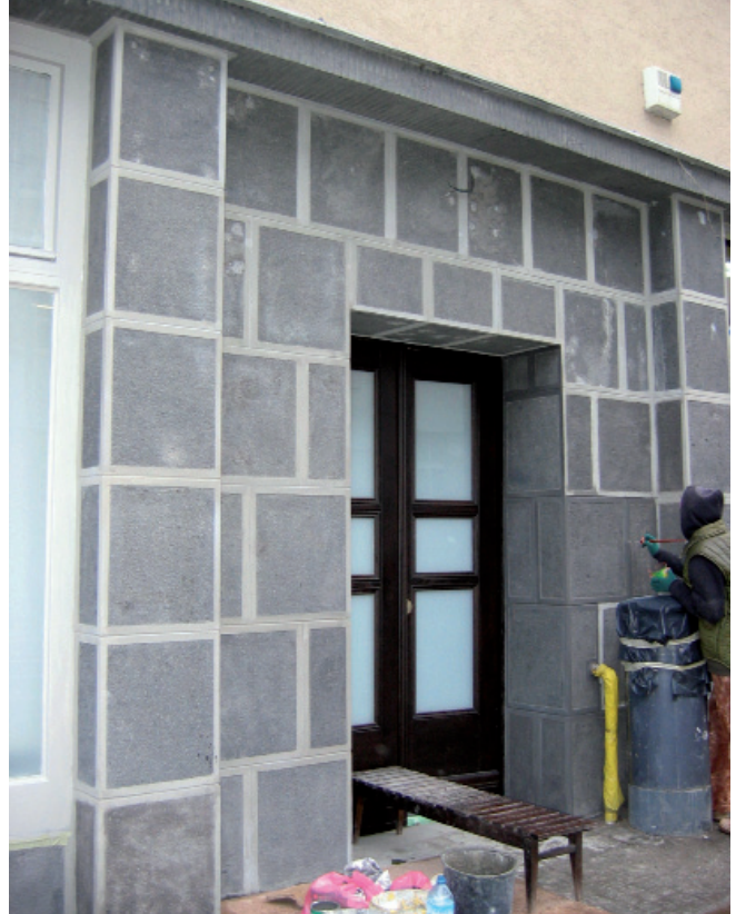
9. Historical plasterwork restoration in the ground floor of 122, Świętojańska tenement. Photo by the author
