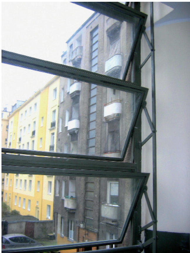
6. Revolving-frame windows of the staircase at 27-31, 3 Maja street after 2007 renovation. Photo by the author
