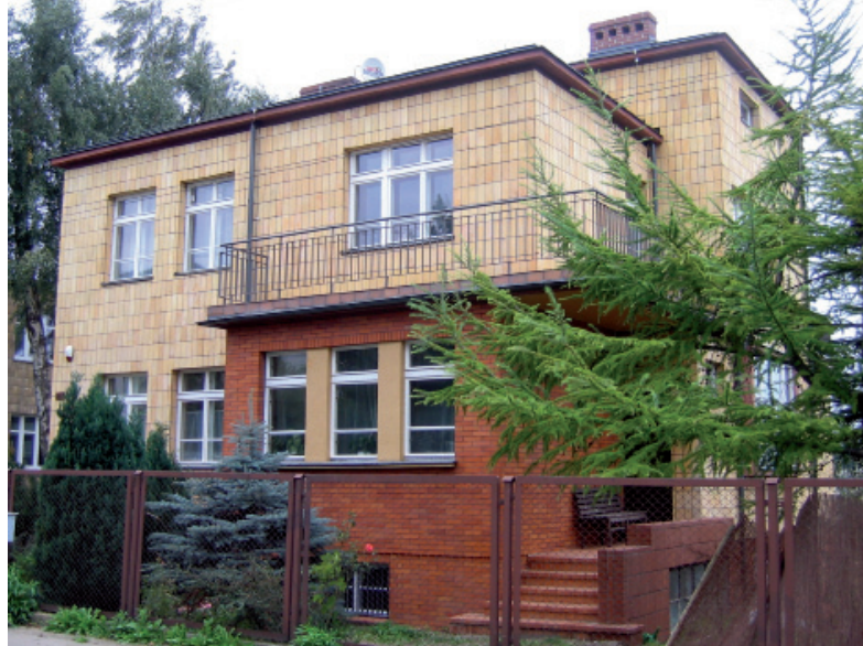
14. Historical villa at 111, Inżynierska after 2007-2008 renovation. Photo by the author
