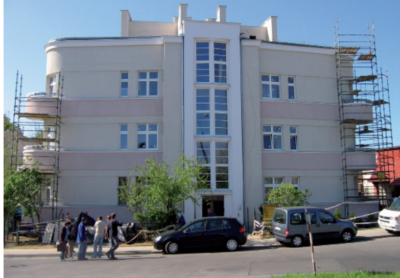
13. "Opolanka" residential building after 2007 restoration. Photo by the author
