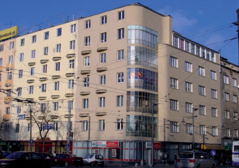
12. A tenement at 122, Świętojańska after 2006-2007 facade restoration. Photo by the author
