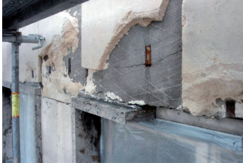
4. The decrepit stone cladding of former FE BGK building at 27-31, 3 Maja street in Gdynia. Photo by the author
